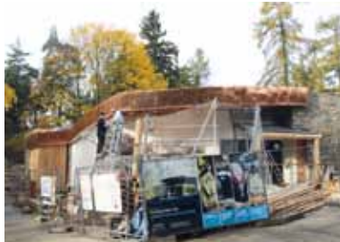
Rozestavěný pavilon Kalahari /Kalahari pavilion during construction/
