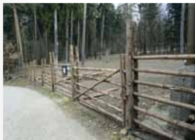
Oprava plotu u sobů /Repair of fencing at the reindeer/
