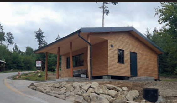
Vybavené kontejnery byly obloženy dřevem /Containers were lined with wood/
